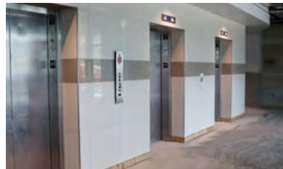
As with much of the new wing's first floor, the elevator lobby is tiled with a light brown marble tile. The ground-level flooring, when completed, will be poured terrazzo.
