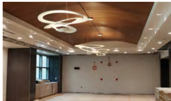
The ceiling treatment in public areas on the first floor, including in this Administration conference room, will feature arched wood.
