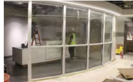
Crews work on the lighting in the Administration reception area.
